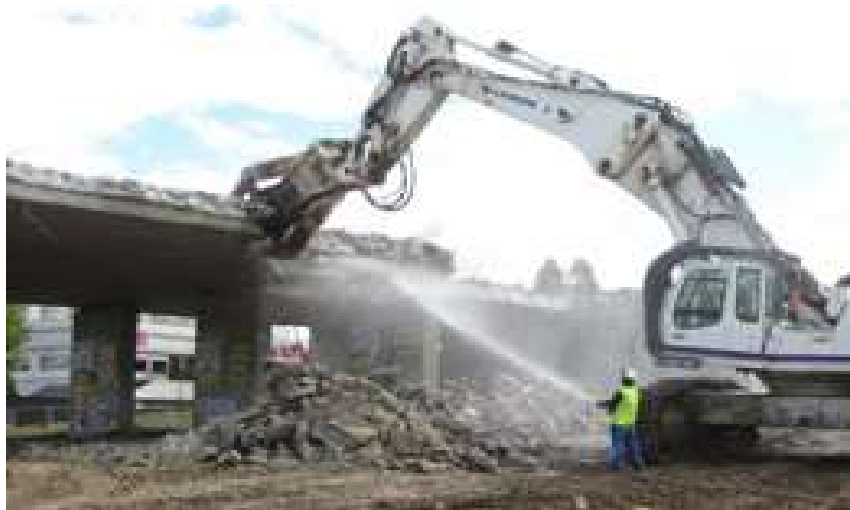
Photo 8: Mechanical shovel deconstruction
