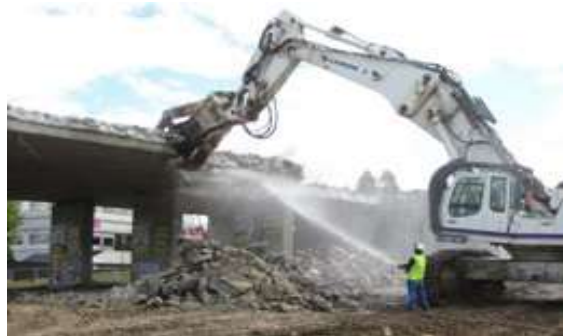
Photo 13: Deconstruction by mechanical shovel
